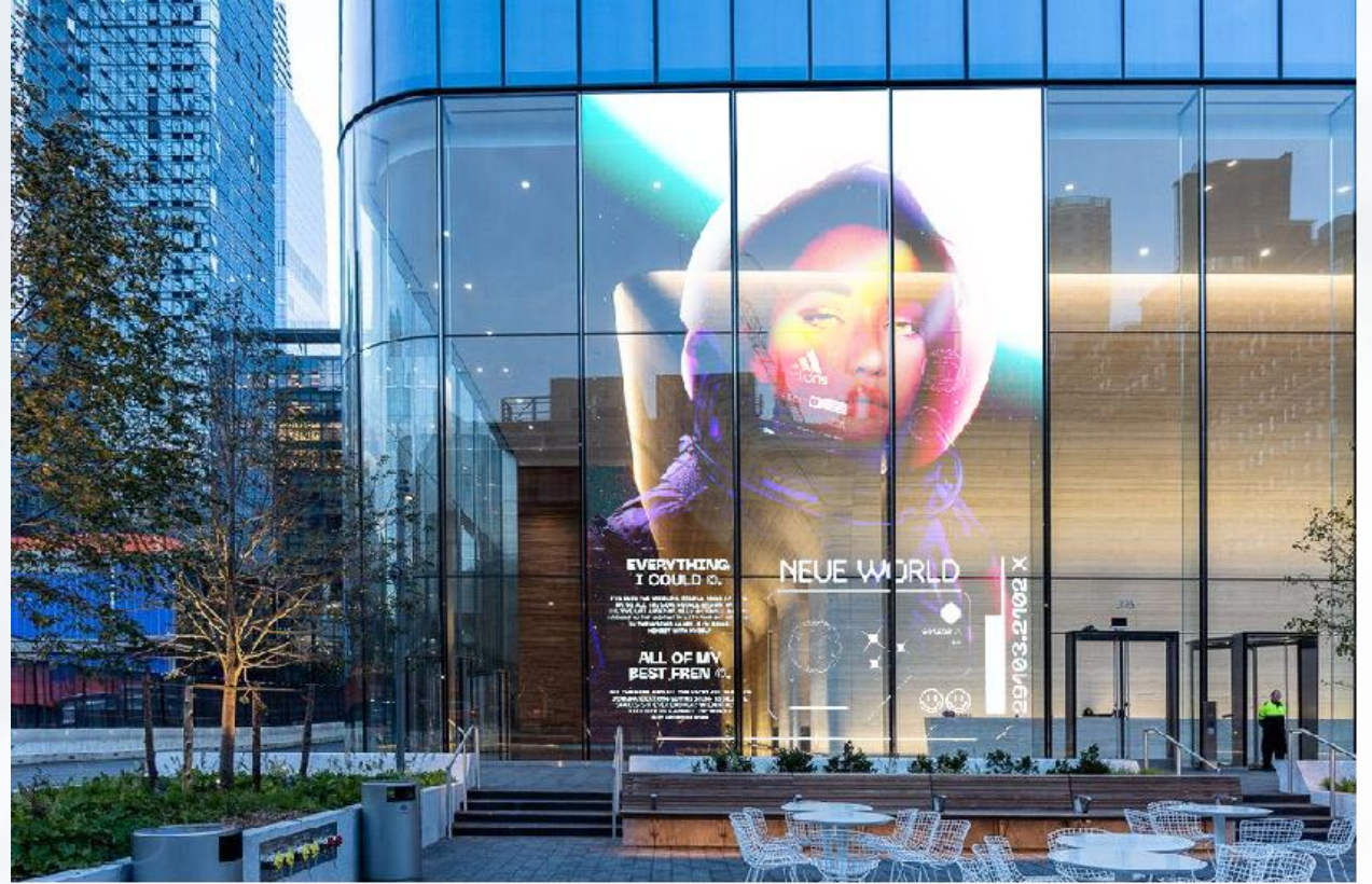
● Building Glass Curtain Wall
